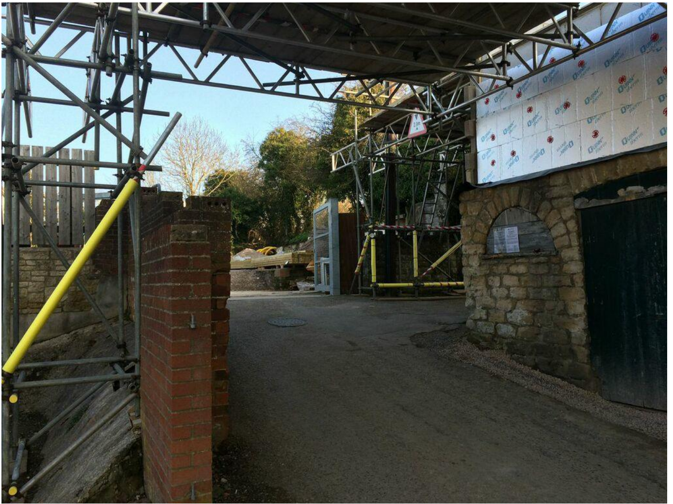
Prospect Place looking further into the site.
