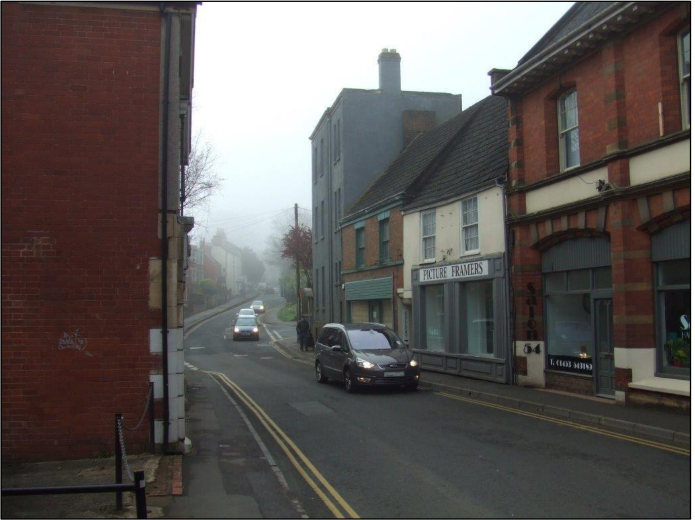
Silver Street, the frontage of numbers 60-54 (view to SW)
