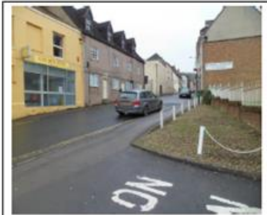
19. Long Street- parking on double yellow lines.
