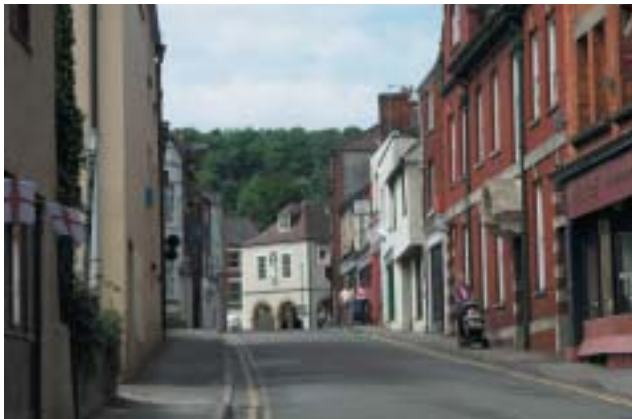
Market Hall is a landmark from several points in the town (example - Silver Street)
