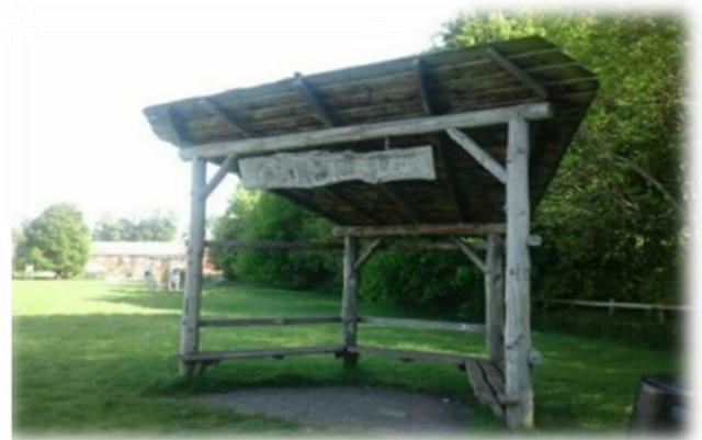
The main wooden support posts had started to rot and a deterioration in the structural condition of the shelter led to its removal. The shelter had been on the site for many years and was installed before we took over management of the site from Stroud District Council.
